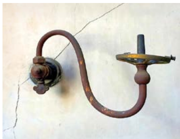
Gas light fixture found on third floor. Electricity wasn't introduced in Raleigh until 1885 and residential use didn't appear until about 1890, meaning the house spent close to two decades without electricity—using gas lights such as this one for illumination.
