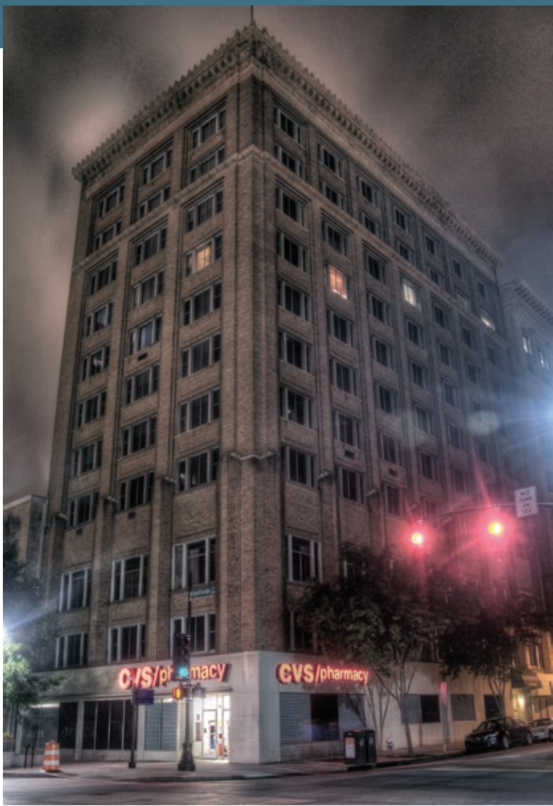
The Raleigh Building in its present day form
