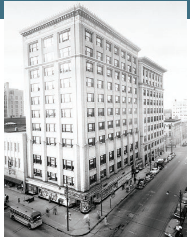
The building in 1940 after the columns were replaced with simple brick piers (ironically a drug store existed at this time in the same spot as the current day CVS).
