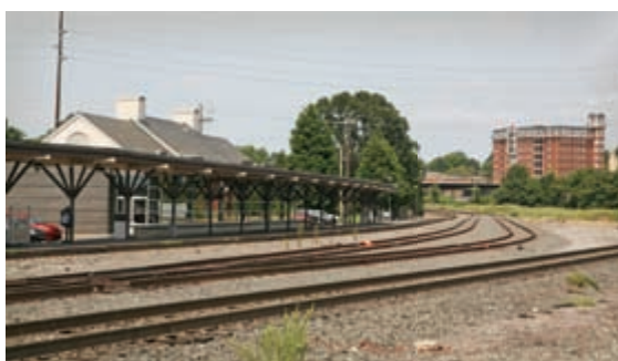
The existing train station between Cabarrus, Davie and Boylan Avenue will be the future home of the multi-modal transit system
