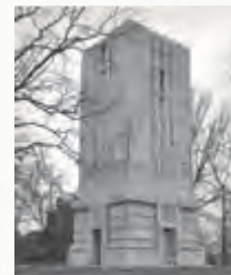
The tower as it appeared for much of the Great Depression, 1930.
