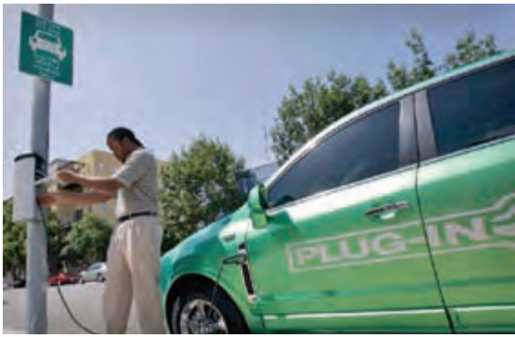
18 city-installed electric vehicle charging stations are available to the public.
