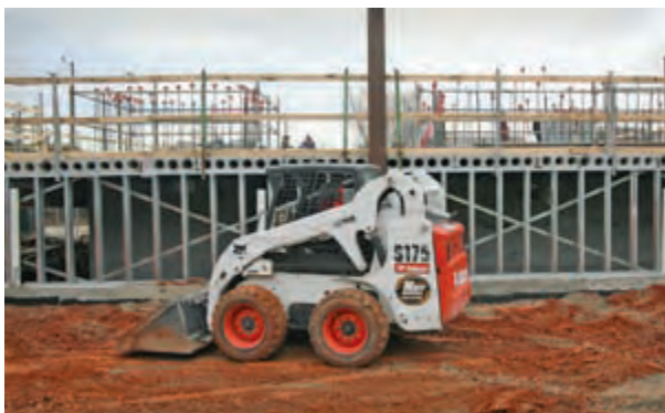
Hampton Inn construction has begun in the new Glenwood South location.
