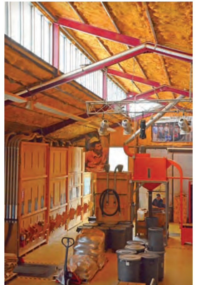
Sunlight-gathering solar clearstory roof inside Larry's Beans' roasting room and warehouse. BY STAFF PHOTOGRAPHER THOMAS M. WAY
