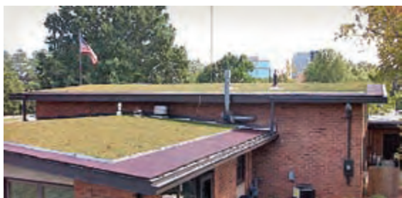
Raleigh Fire Station 9 has sported a green roof since 2009.
