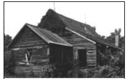
Just north of downtown, this building is believed to have been the last remains of Isaac Hunter's Tavern. It remained standing until the 1970s.
